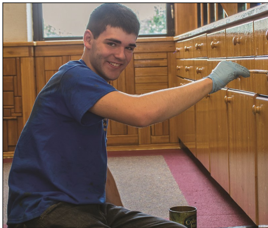
Junior Jake Ziede applies polyurethane to the wooden cabinets
