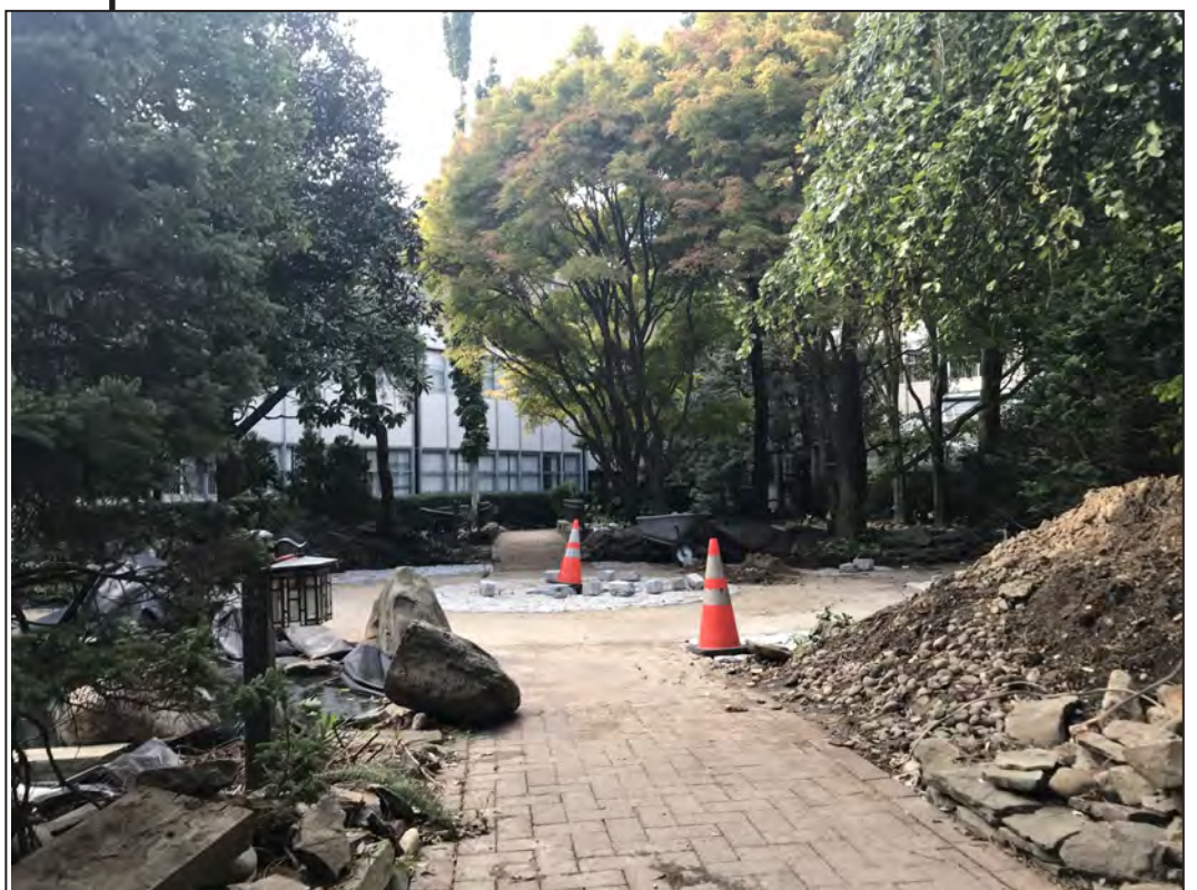
Above, the new expanded center circle walkway of the courtyard can be seen under renovation.
